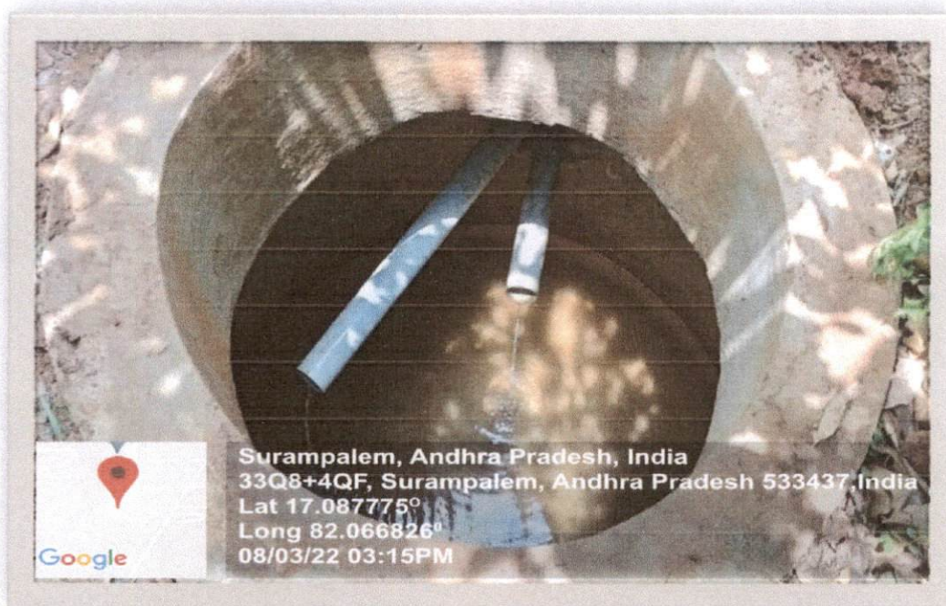
Treated Water Collecting Tank
